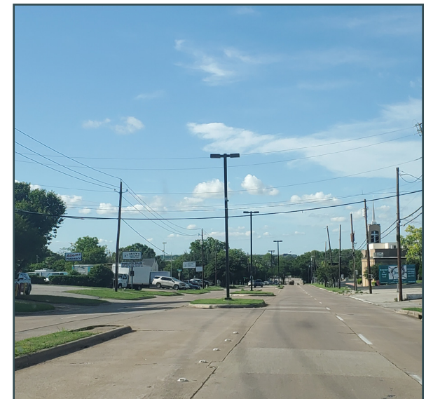
Raised Medians break up the center turn lane
