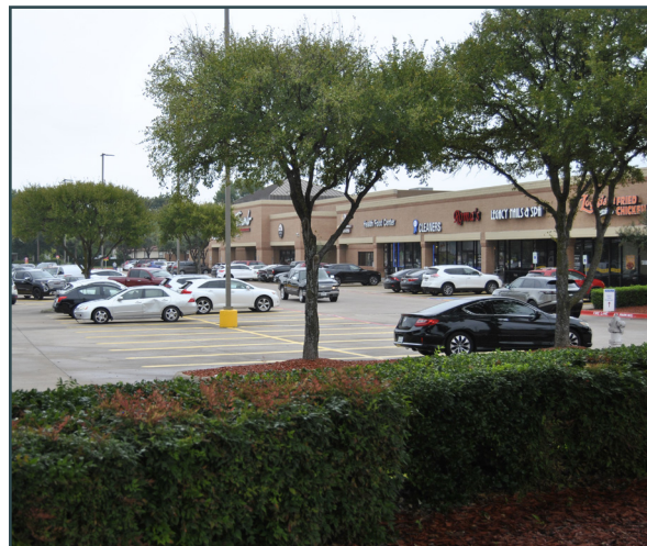
Strip Commercial Center
