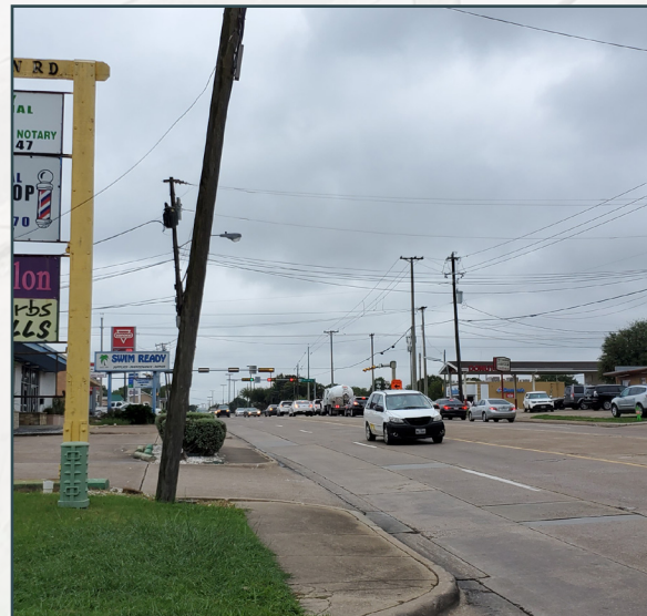
Utility lines exist along Hampton Road
