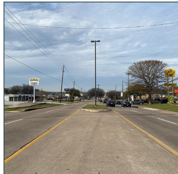
Five Lane Roadway Conditions
